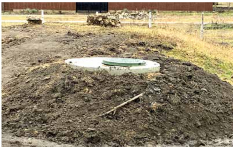
■ Das Wasserreservoir in Bahu.
